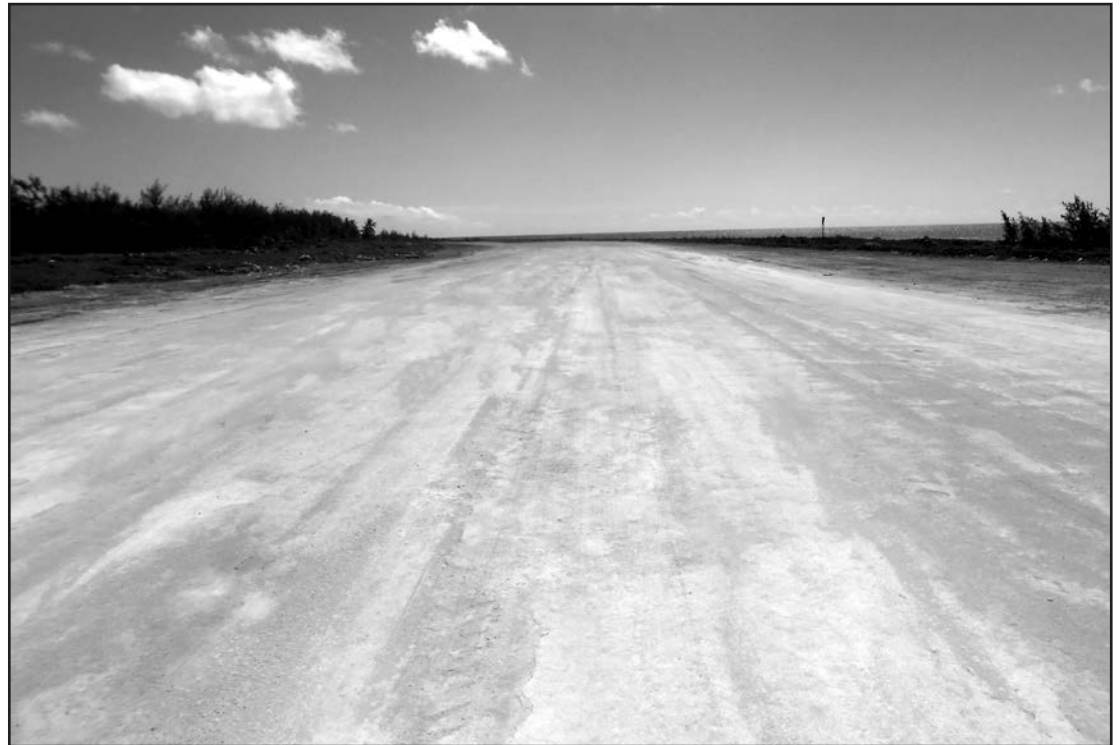
Mitiaro airport runway with upgrading completed.
